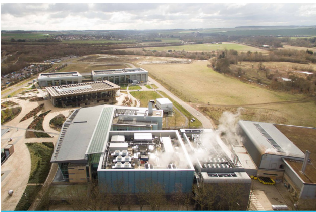
Wellcome Trust: Data Centre 4th Quadrant ■ £10m NEC3
